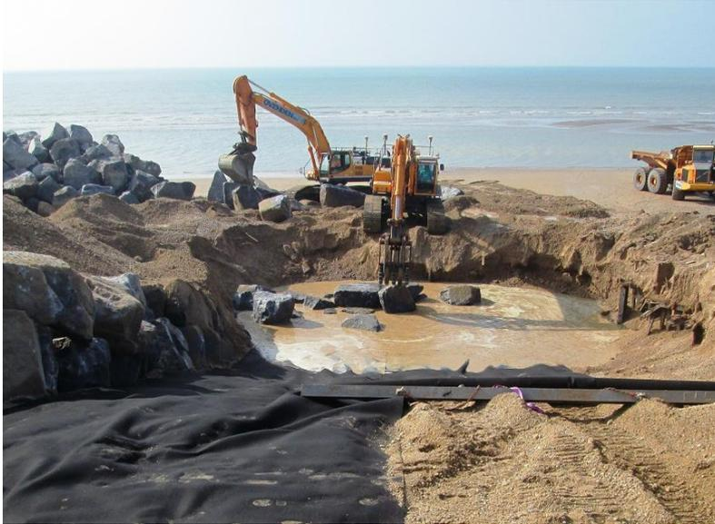
It is anticipated that virtually all deliveries will be made from the sea and will not be brought through the village. Construction of the rock berm can only take place at low tide and in order to progress the works quickly we may work early in the morning or in the evening, to maintain the momentum of the project and complete it before the
