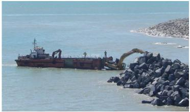
The rock placing machines are fitted with the latest Gobal Positioning System (GPS) technology, with a computer which screen shows the operative a virtual model of the rock berm. This allows for and accurate speedy placement of the rocks.
