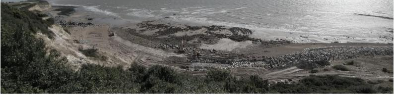
Aided by the good weather, progress has been excellent and the works are now approximately 85% complete. The construction process has attempted to blend together the stage 3 berm with the two existing berms, as you see from the photographs and on the ground. We also intend to carry out some maintenance of the two existing berms where necessary while we are on site. This is work that will strengthen both existing berms.
